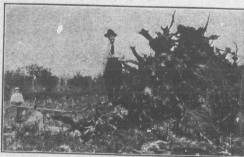
Clearing Land With a Hand Stump-puller.
