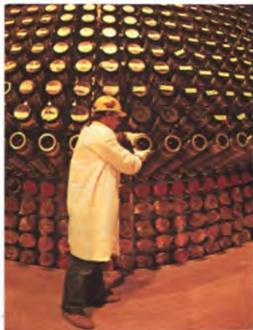
Part of the CANDU reactor system at Pickering, Ontario. Each of the 390 pressure tubes holds 12 fuel bundles.
