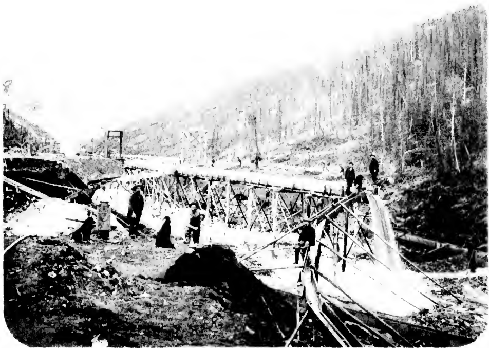
BRIDGE UNDER CONSTRUCTION
