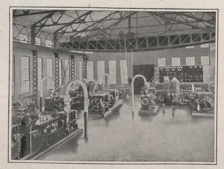
EACH CORLISS UNIT 20 & 40 x 36, DIRECT CONNECTED WE BUILD:
