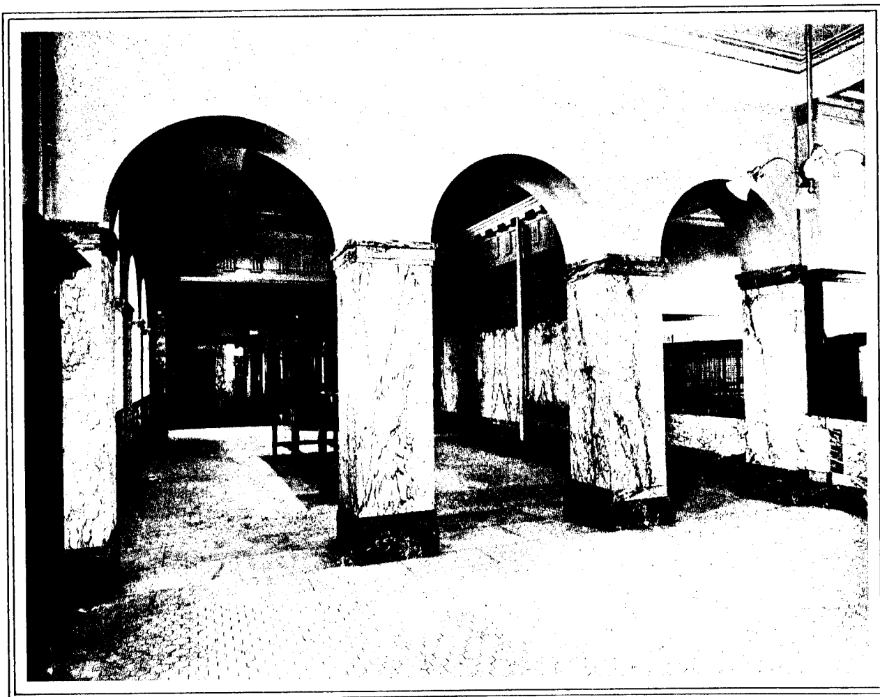
Section of Interior of Customs House, Toronto, Showing Marble Work Executed by Us.
