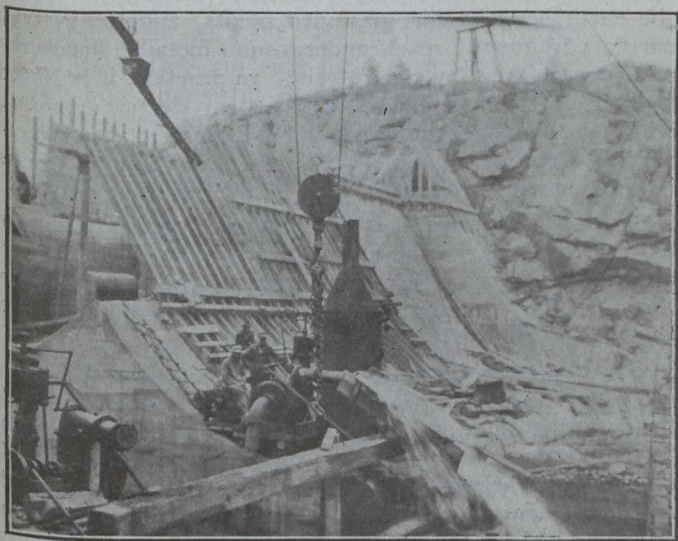
Fig. 4.—Pumping Out Sluice Pipe Chamber Preparatory to Connecting Sluice Pipe with Sluice Valves
