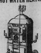
Water circulation completely surounded by fire, resulting in great heatng capacity with small fuel consump-
