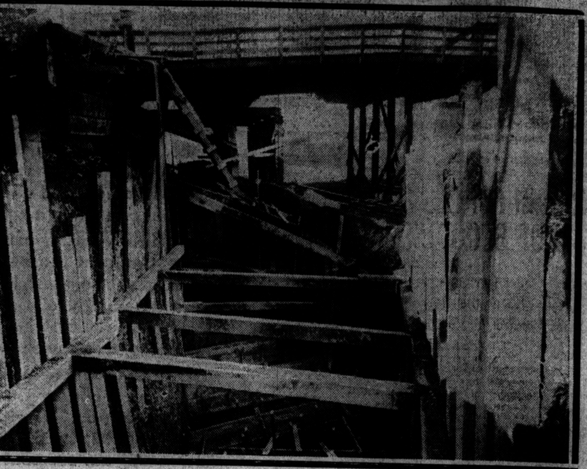
The old bridge across the Grand Trunk tracks at Strachan avenue, shown in the upper photograph, must be demolished. A new bridge will be built twelve feet higher. It will form a new motor drive to the Exhibition, will be 60 feet wide and 92 feet long. The lower photograph shows the piling for a cement sewer 18 feet wide, which will be built alongside the new bridge.
