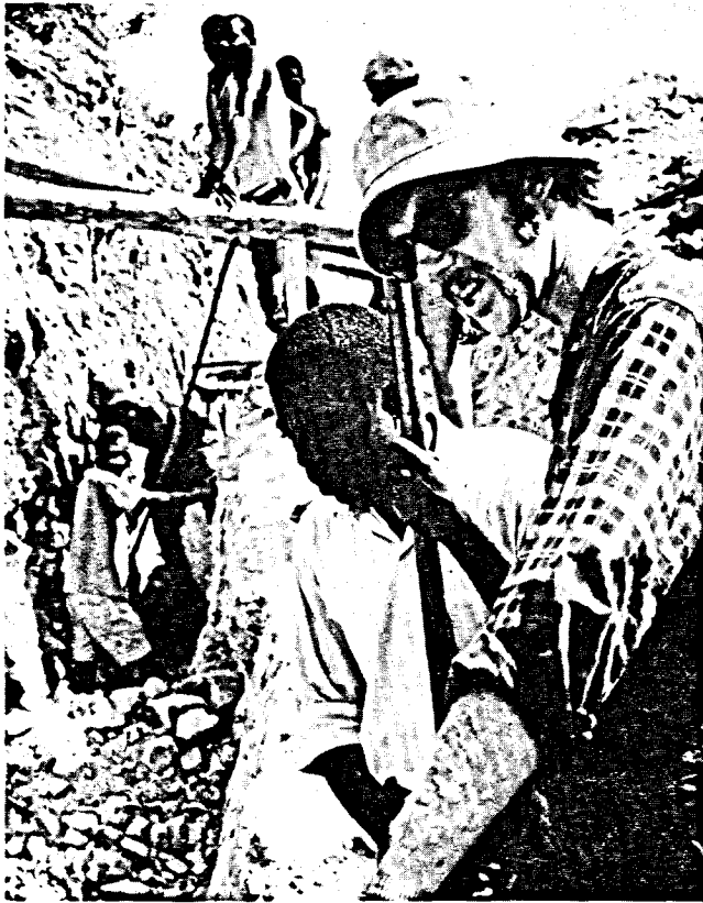
John Campbell, a civil engineer from Richmond Hill, Ontario, employed by CIDA, supervises the construction of a sewage system in Blantyre, Malawi.
