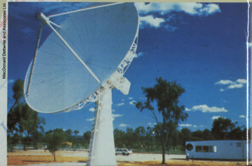
The LANDSAT tracking antenna and reception laboratory installed at Alice Springs, Australia, is an example of MacDonald Dettwiler's complete turnkey service.
