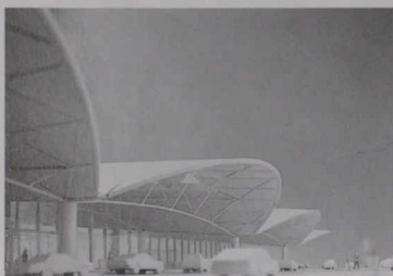
A landside view of the terminal complex. The building will have a unifying modular roof structure made primarily of steel.
