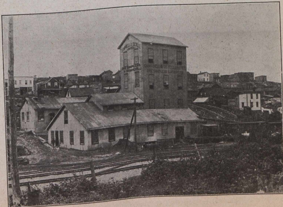
General View of Plant.
