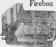
Durability in a firebox depends mostly upon its ability to expand when hot and to contract when cold, without cracking.
