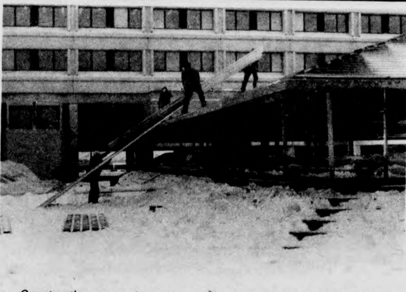
Construction proceeds on new religious centre atop Central Square.
