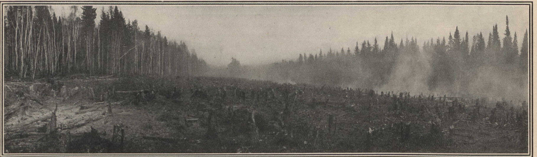
Clearing the right of way of the Junction of the Temiskaming and Northern Ontario Railway with the National Transcontinental, and laying out the Town of Cochrane. Since this photograph was taken, about October 1st, some buildings have been erected and some of the streets graded.
