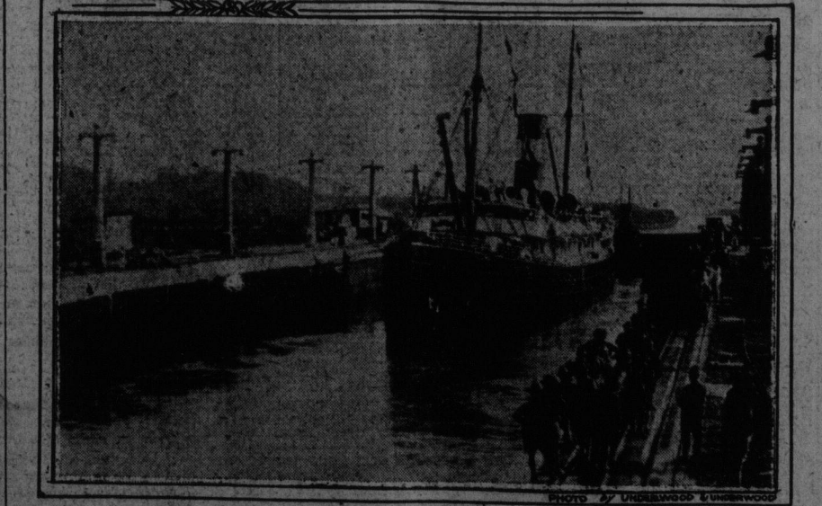
The steamship Alliance, belonging to the Panama Railroad Company, is the first large vessel to pass through the Gatun locks of the Panama Canal. It was on June 9 that she was sent through the locks for the purpose of testing the electric locomotives that will be used to tow vessels through the locks. The test was a success, the locomotives handling the four thousand ton steamship easily and speedily. It took the Alliance one and one-half hours to pass through the locks.
