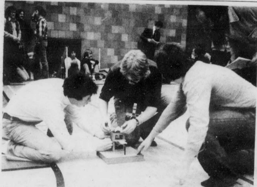
Twenty-five square feet of plastic, four square feet of masonite, two elastic bands, a mouse trap and twine were all the second year Mechanical Engineers had to work with in their Annual Design Contest. This year's task involved the design and production of a flying mechanism which would maximize air time. Winning time was about 3 1/4 sec.
