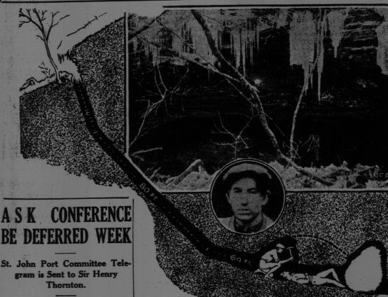
Above is entrance to Sand Cave, near Cave City, Ky., where Floyd Colions was trapped by an 18-ton boulder which dropped from the roof, plining his foot. Diagram shows how Collins was trapped. Dotted line is where workers hoped to clear space to free Collins, but a series of cave-ins shut off this passage. They are now driving a new shaft from ground level directly behind the stricken man. Smaller inset is Jewel Este, 17, who discovered Collins' plight.
