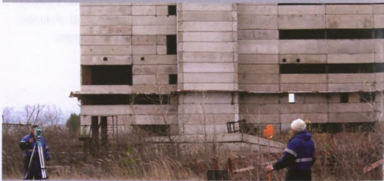
Canada has contributed $9 million to the U.S.-led project to shut down the last Russian weapons-grade plutonium-producing reactor, in Zheleznogorsk. This reactor produces enough plutonium for approximately one nuclear bomb per week. Photo Credit: US Department of Energy (DOE)
