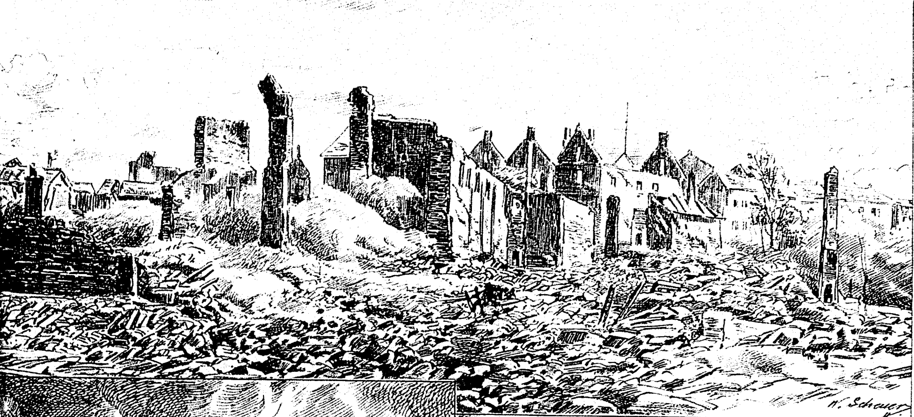
ET, FROM THE CANAL, AFTER THE FIRE.
