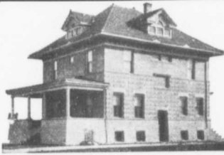
Note the Artistic Effect of "Ideal" Blocks in Residence Construction.
