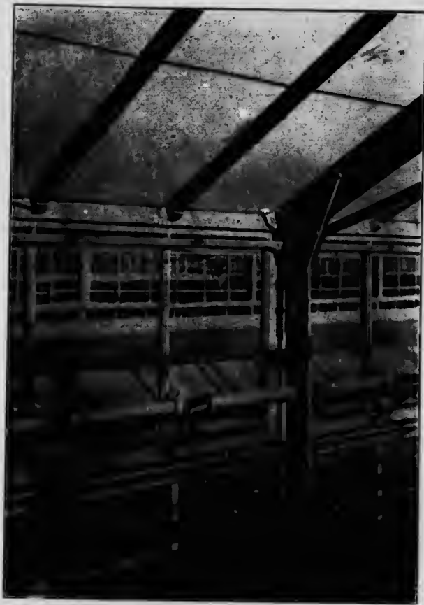
Iron frame construction—showing the iron member which acts as the supporting part of the house. Solidity is the feature here.
