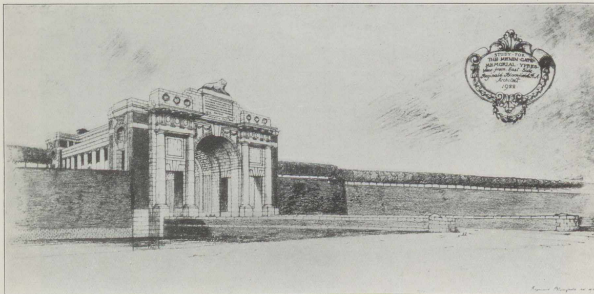
HALL OF MEMORY. MENIN GATE. IN COURSE OF ERECTION BY WAR GRAVES COMMISSION.
