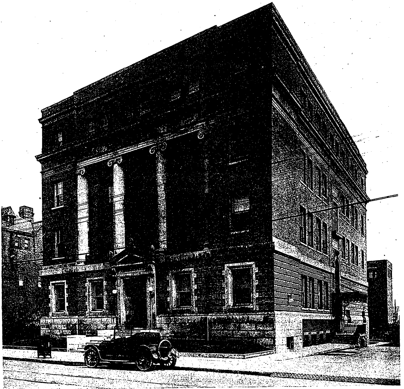
BOARD OF EDUCATION ADMINISTRATION BUILDING, TORONTO.
