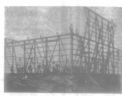
Photo No. 2—Shows, in course of construction, one of the largest "Steel Truss Barns" ever built. Only a few men are visible in this view—and as a matter of actual fact, but 14 men were employed in its construction. This barn was built for Mr. Conrad Gies, St. Clements, Ont.
