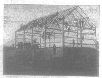
Photo No. 1—Reproduced above, shows a typical barn raising, on a farm in Lambton County, Ontario. This is one of the old-fashioned timber frame barns—and though it is a comparatively small building, the photo reveals that there were exactly 39 men engaged on this job.
