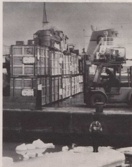
In mid-August, barges with prefabricated housing components are unloaded on the ice-rimmed shore of Holman Island.
