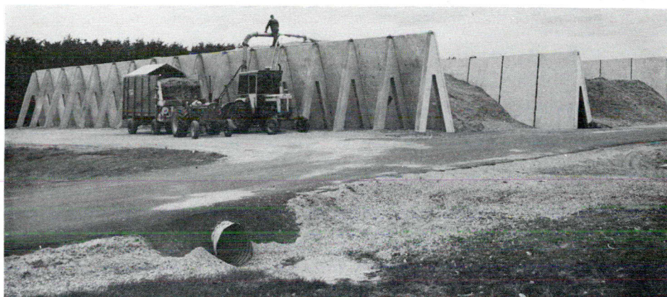
Agriculture Canada employees filling the two new concrete horizontal silos
