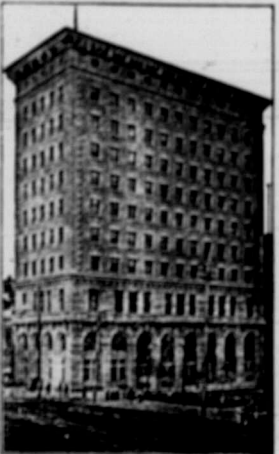
Union Bank Building, Winnipeg
