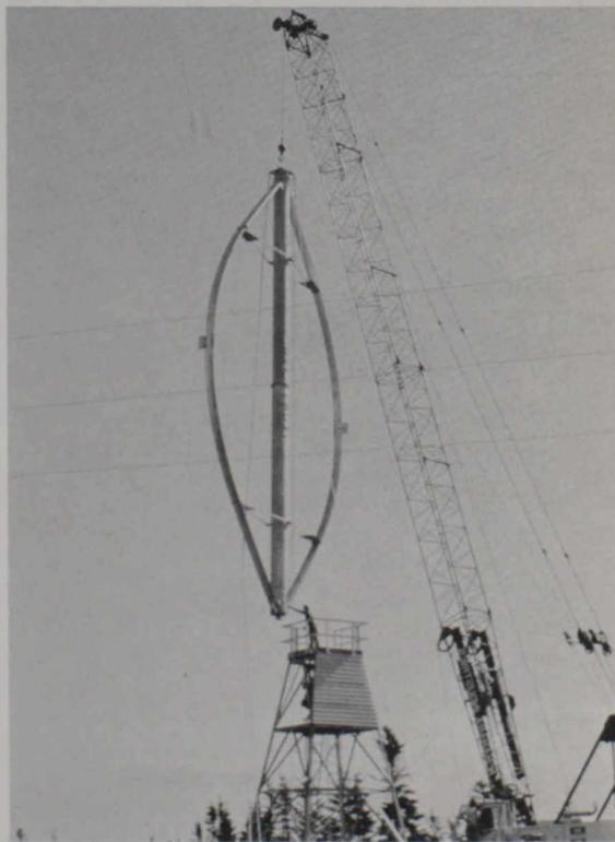
*Small and medium sized windmills can serve specific household or industrial purposes. This middling one, producing 55 kilowatts, generates electricity which is fed into the hydroelectric grid in Newfoundland.*
