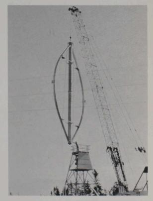
Small and medium sized windmills can serve specific household or industrial purposes. This middling one, producing 55 kilowatts, generates electricity which is fed into the hydroelectric grid in Newfoundland.
