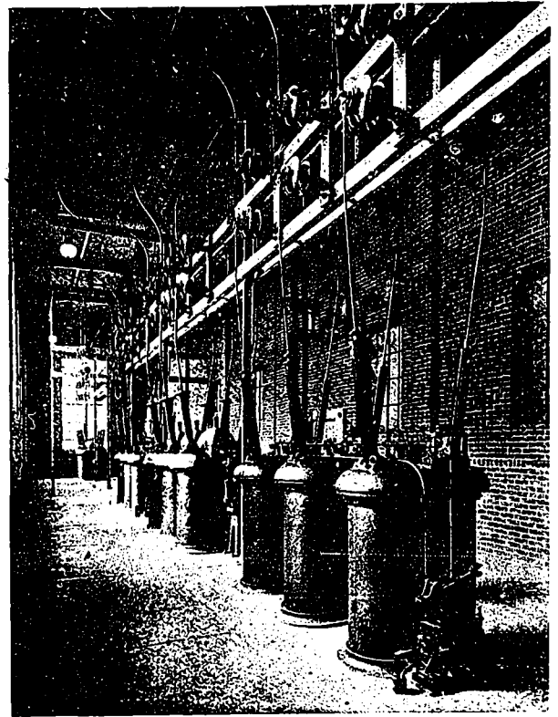
OIL SWITCHES AND BUSES FOR 42,000 VOLT CURRENT.
