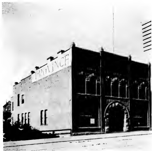
"THE PROVINCE" BUILDING, VANCOUVER, B.C.
