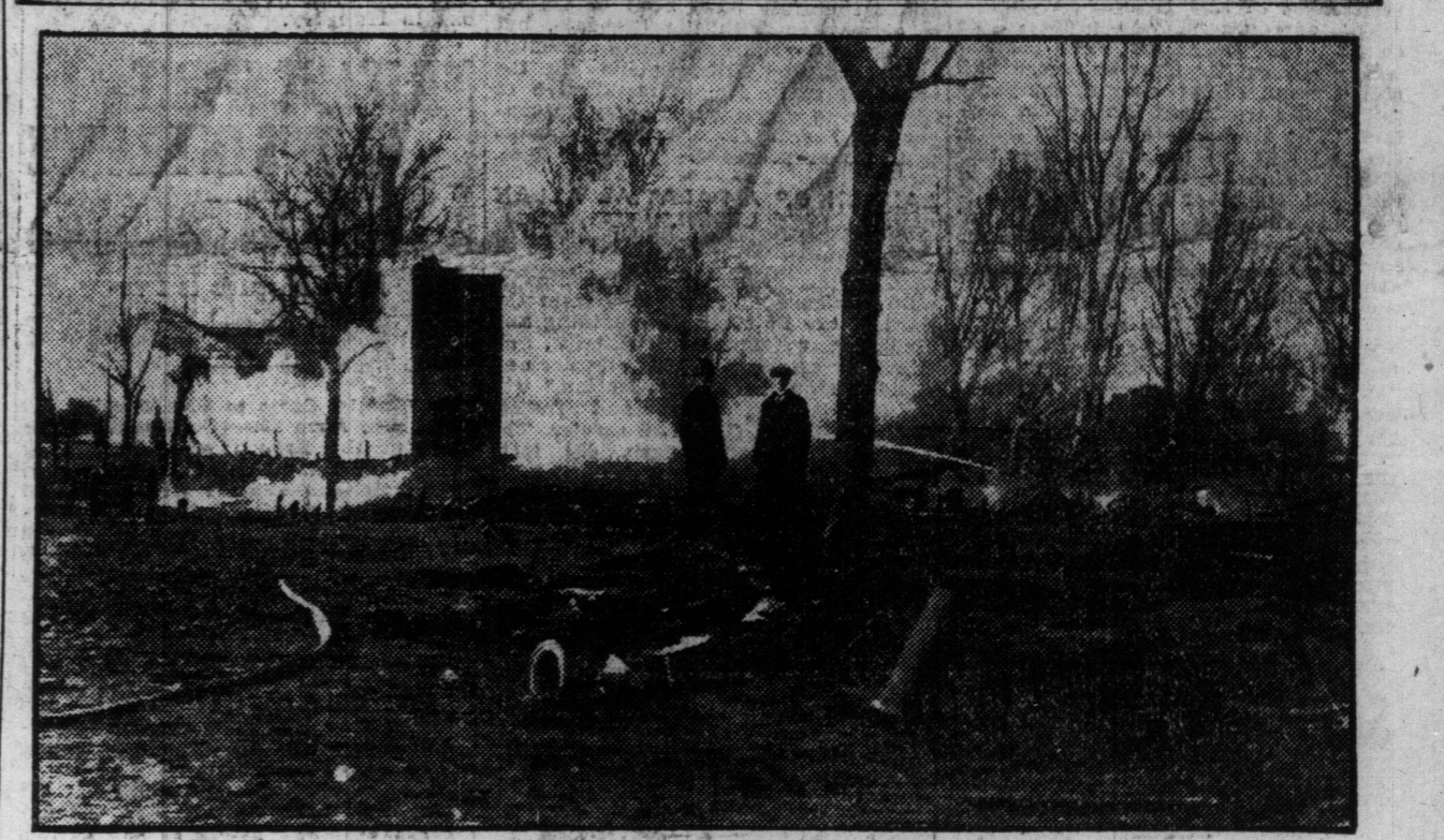
The Fire Boat's Hose Playing on the Smoking Ruins of Mrs. Horwood's 30-Room Boarding House. Each of the Six Houses Was Reduced to Ashes.
