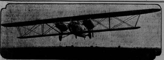
THE great triple-motored Sikorsky plane in which Capt. Rene Fonck and his companions plan to make their non-stop flight from New York to Paris here is shown in test flight at Roosevelt Field, Long Island. The wings have a spread of 150 feet across, and the plane will carry a load of 25,000 pounds.
