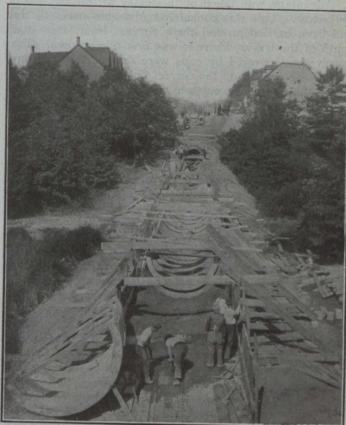
Illustrating Open Cut and Method of Construction
