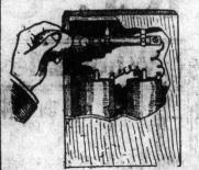
been invented, utilizing electric ligh. The current is generated by dry bat eries and the tester is easily carried the hands. It has an opening of one side that is partly closed by pring. The egg to be tested is pres ed hard against this opening. Th pring slips aside and permits the eg. to be forced into the hole where i can be examined through the light.
