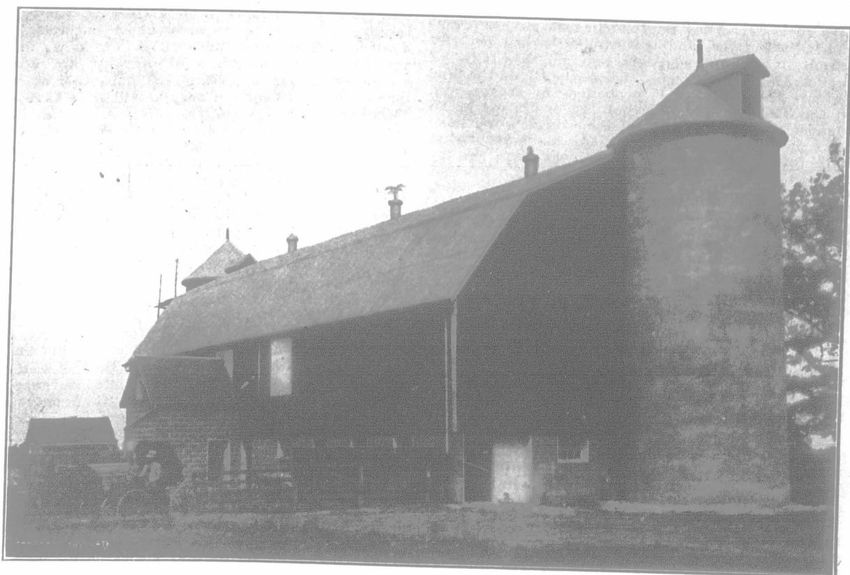
An Elgin County Dairy Barn.
