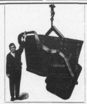
BECAUSE they are so designed that the "Tilting-Bottom device" deposits concrete, sand, rock and other materials in ONE PLACE with ONE upward pull of the handle and ONE MAN to operate.
