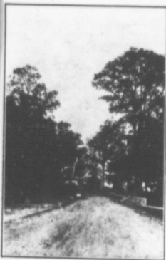
Cut No. 85 Building Protecting Walls Around Trees.
