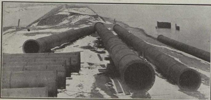
Fig. 6.—Sections of Beach Intake Pipe Before Placing.
