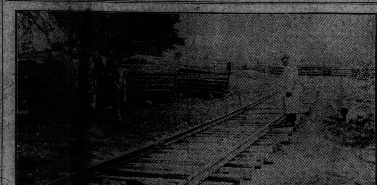
Ties and Timbers Brought into Port Weller Over a Spur Line From the New C.N.R. Electric Road From St. Catharines to Niagara-on-the-Lake.
