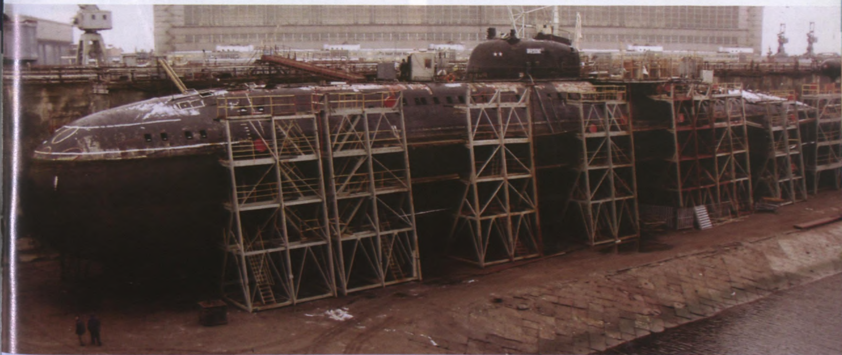
Victor III being dismantled in dry dock
