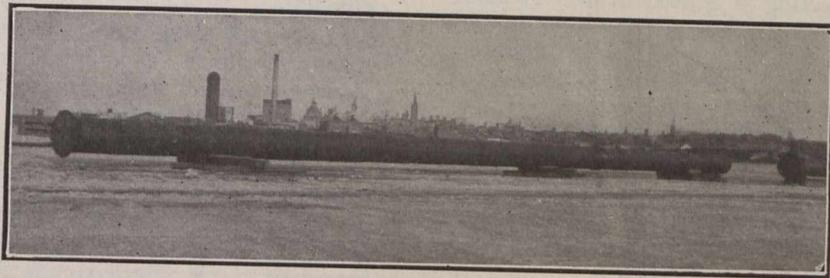
Fig. 1.—A Length of Pipe Ready for Relaying
