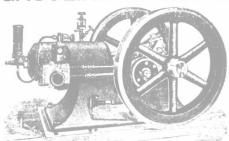
For grinding, sawing, pumping and threshing purposes. Portable and stationary. Made by Goldie & McCulloch Co., Galt. THE BURRIDGE CO., Agents, WINNIPEG.
