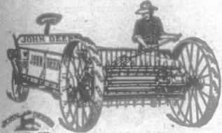
Take any manure spreader you have ever seen, remove all the clutches and chains, all the countershafts and stub axles, do away with all adjustments and mount the beater on the rear axle.
