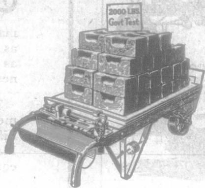
**Exacting Tests—Every Renfrew Truck Scale is tested by a government inspector in our factory. The pictures show some of these exacting tests. Not only do these tests include those for various weights up to 2,000 pounds, but for correct weighing on sides, ends and corners. Every Renfrew carries a government certificate of correct weight.**
