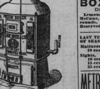
Water circu'ation completely sur rounded by fire, resulting in great heat ing capacity with small fuel consump
