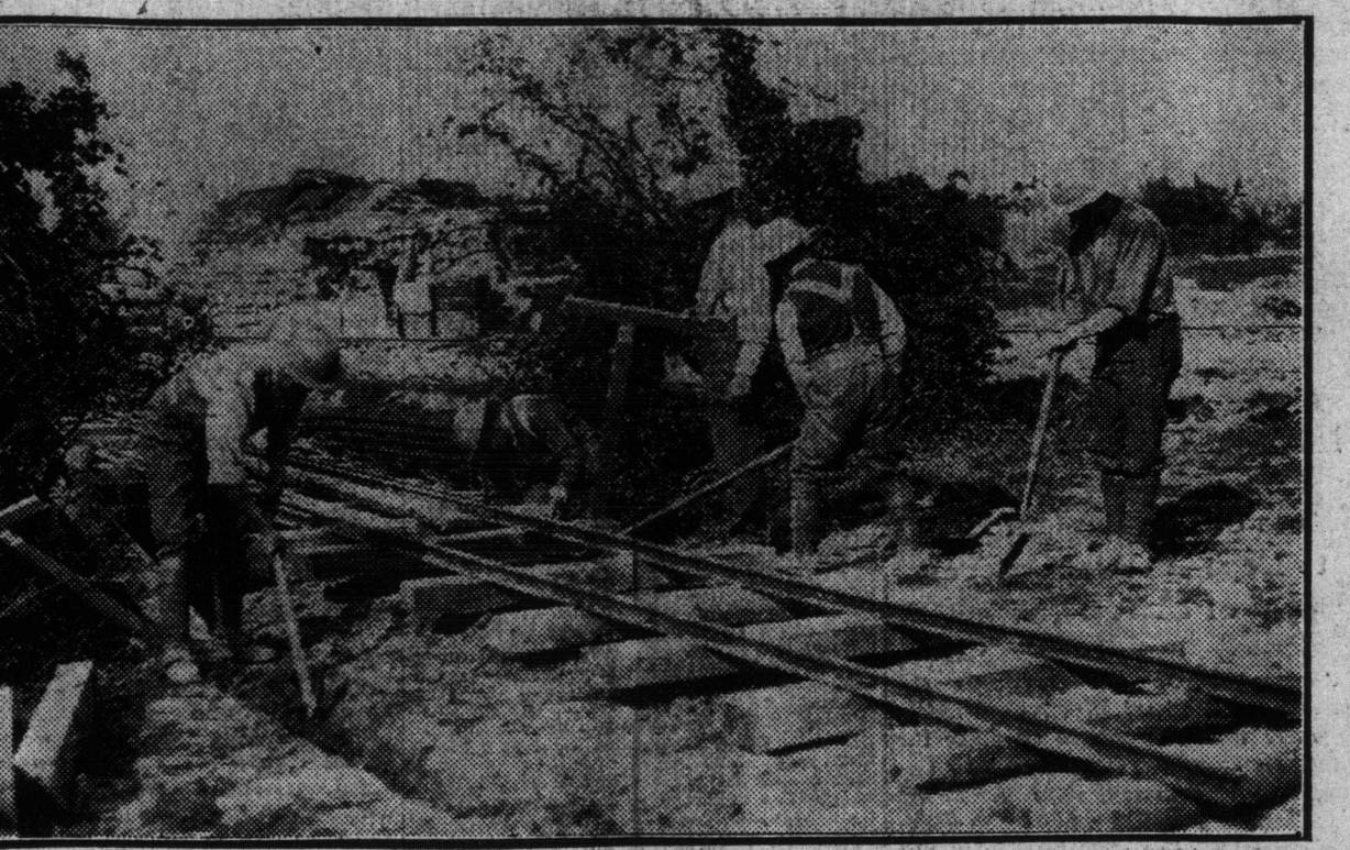
CANADIAN OFFICIAL PHOTOGRAPH FROM THE WESTERN FRONT. Canadian railway troops, working in shelled area, laying track, which will end within a few hundred yards of enemy trenches.
