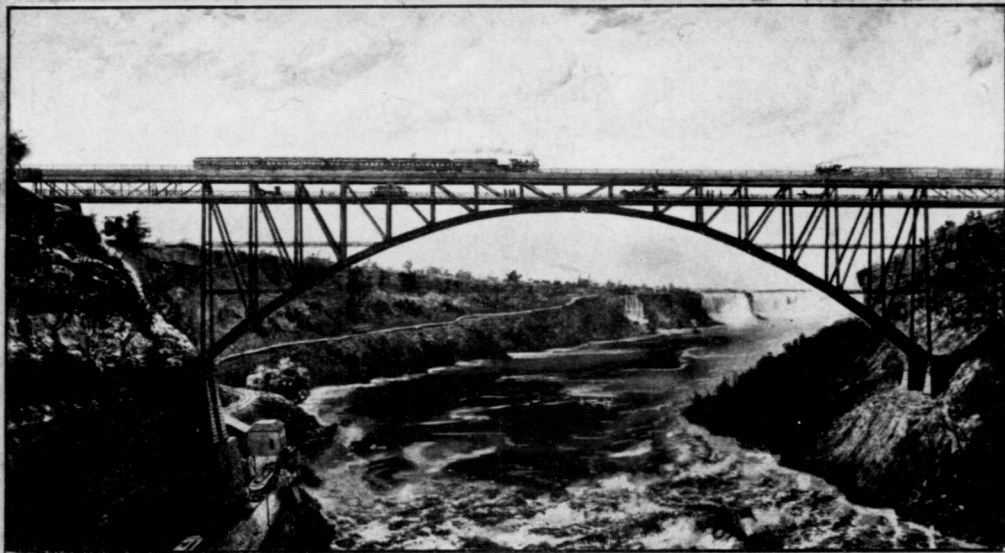
GRAND TRUNK NEW SINGLE-ARCH DOUBLE-TRACK STEEL BRIDGE OVER THE NIAGARA RIVER.
