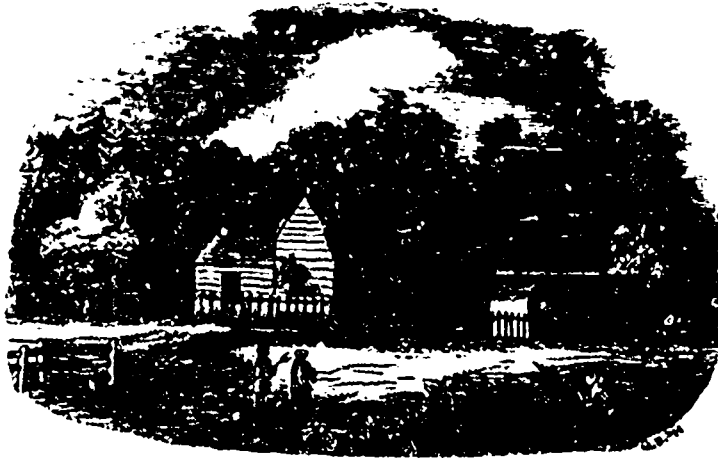
JOHN JONES HOUSE AT THE CREDIT, WHERE DR. RYERSON RESIDES.
